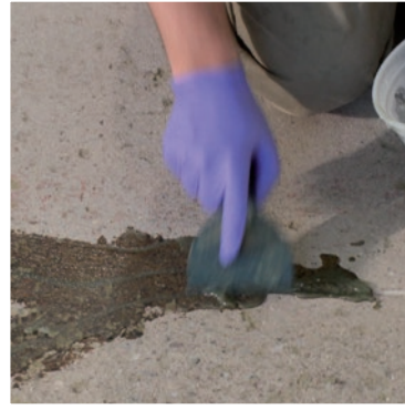
CRACK REPAIR
